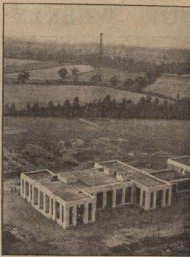
The new London station at Brookman's Park.
